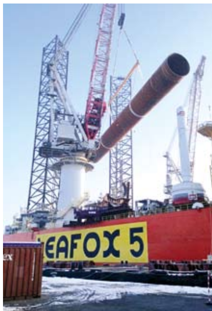
Loading a 700 tonne monopile onto Seafox 5
