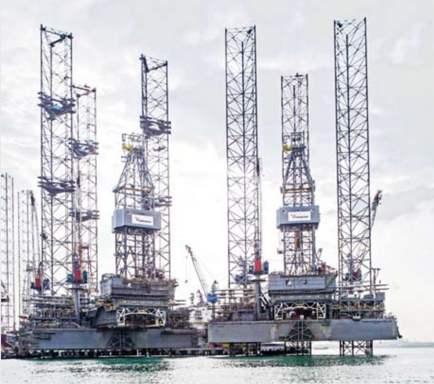
With four KFELS B Class/Super B Class rigs delivered this year and another 16 on order, the design is today the industry standard for modern jackup rigs
