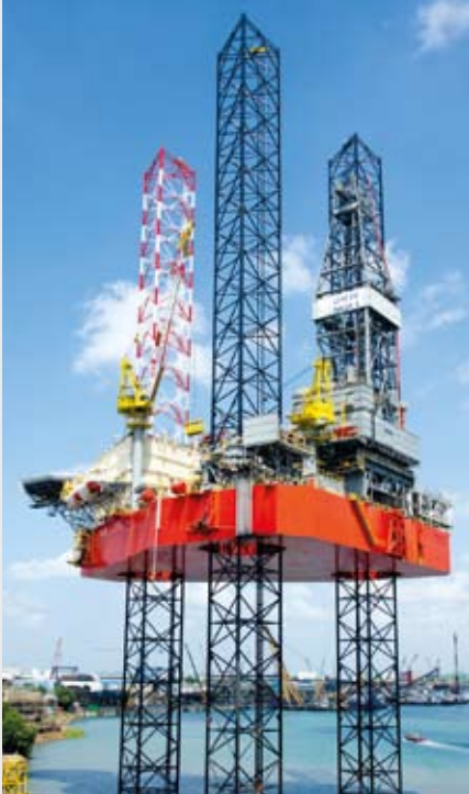
UMW NAGA 4 was completed five days ahead of schedule, on budget and with a perfect safety record for UMW Oil & Gas Corporation Sdn. Bhd
